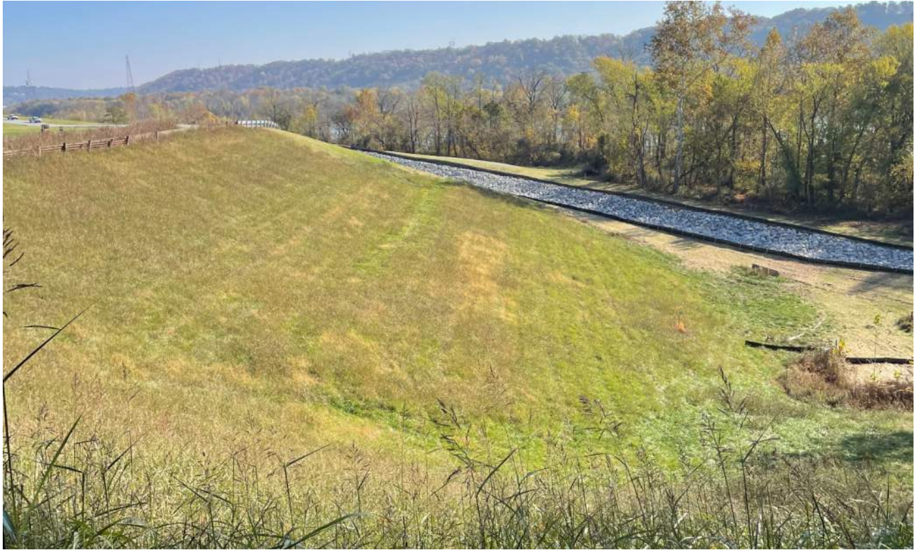
Photograph 1 – West downstream side of LRCP looking east.
