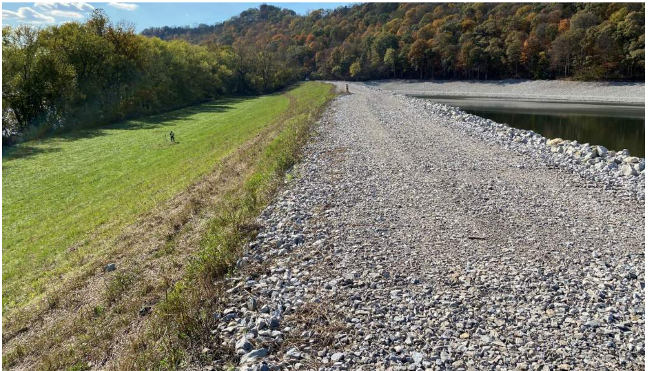
Photograph 4 – South dike embankment crest, looking west. Note the brown damaged vegetation parallel to the top of the slope.
