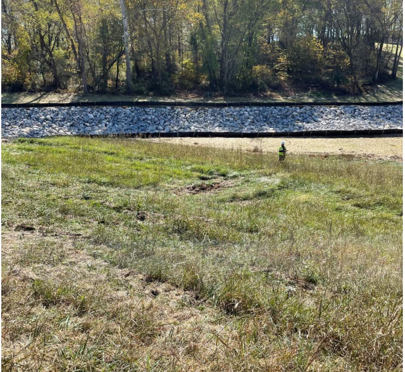
Photograph 9 – Western downstream side where the channel extends along the face and toe of the embankment. Note disturbed spots in grass from equipment.
