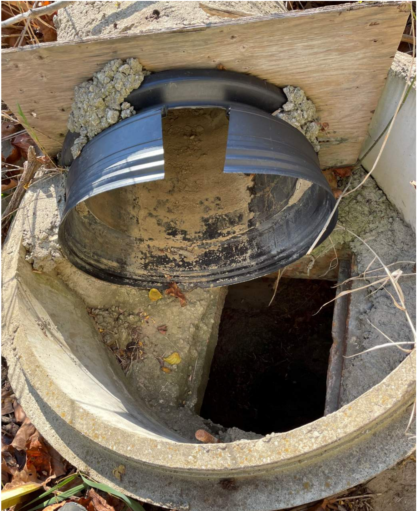
Photograph 8 – Current inlet structure for Outfall 001.
