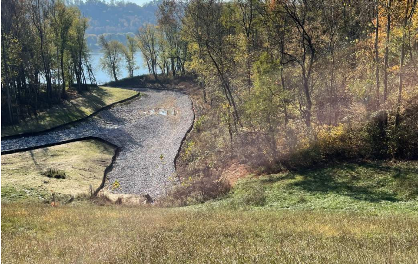
Photograph 3 – Downstream side of dam, newly constructed outfall channel to the Ohio River.
