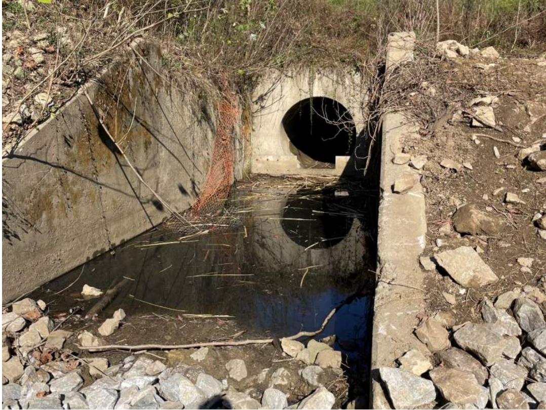
Photograph 5 – Outfall 001 outlet structure at toe of dam.
