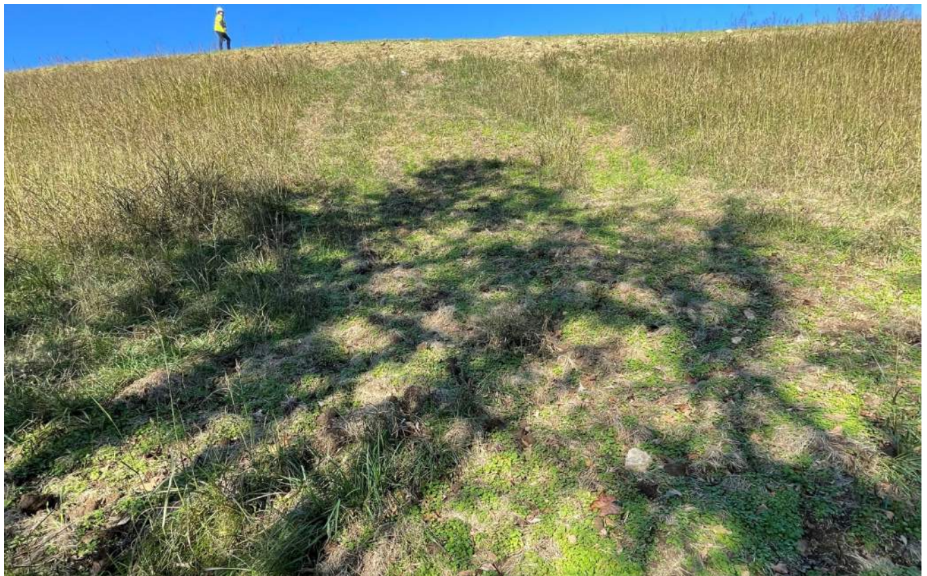
Photograph 13 – Downstream side of dam east of access road. Several areas of sparse vegetation where the bulldozer traversed the slope.
